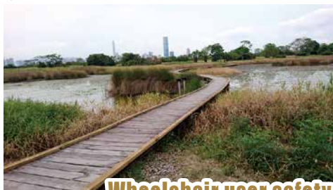
▼ After the installation wood kerbs on boardwalk
