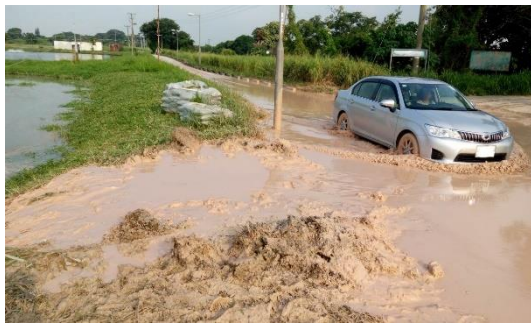
Figure 3. Slurry from the underground pressurized TBM excavation chamber leaked to aboveground through a plugged borehole, which flooded the Tam Kon Chau Road, damaged the structure of the affected fishpond and caused potential adverse ecological impacts on the nearby wetlands.
